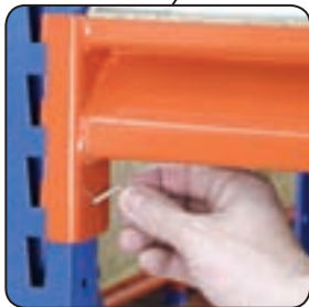
Secure location of beams
